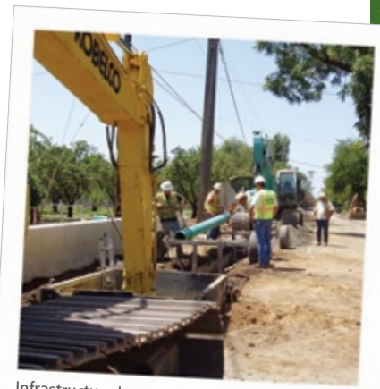
Infrastructure Improvement Project
